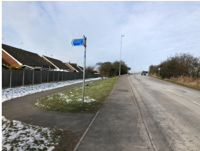
Photograph 5: The 'spur' connection off Eakring Road leading to the National Cycleway.
