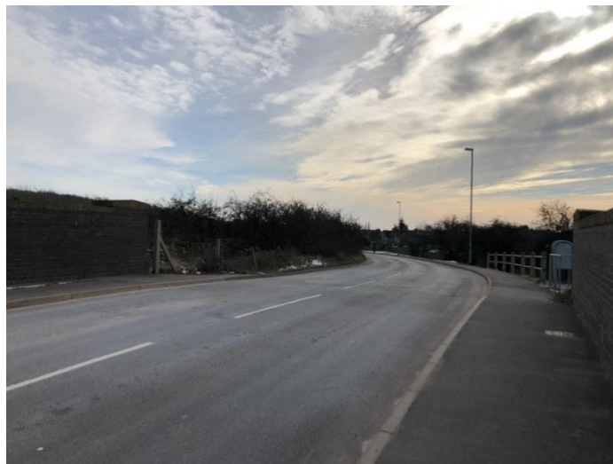
Photograph 12: The views across the site are largely obscured by the brick walls of the bridge. The wide carriageway and gentle sweeping curve of Eakring Road allows higher speeds than the signed 30mph limit. The design of the road offers visual cues to drivers that suggests a higher speed road (looking in a southerly direction).
